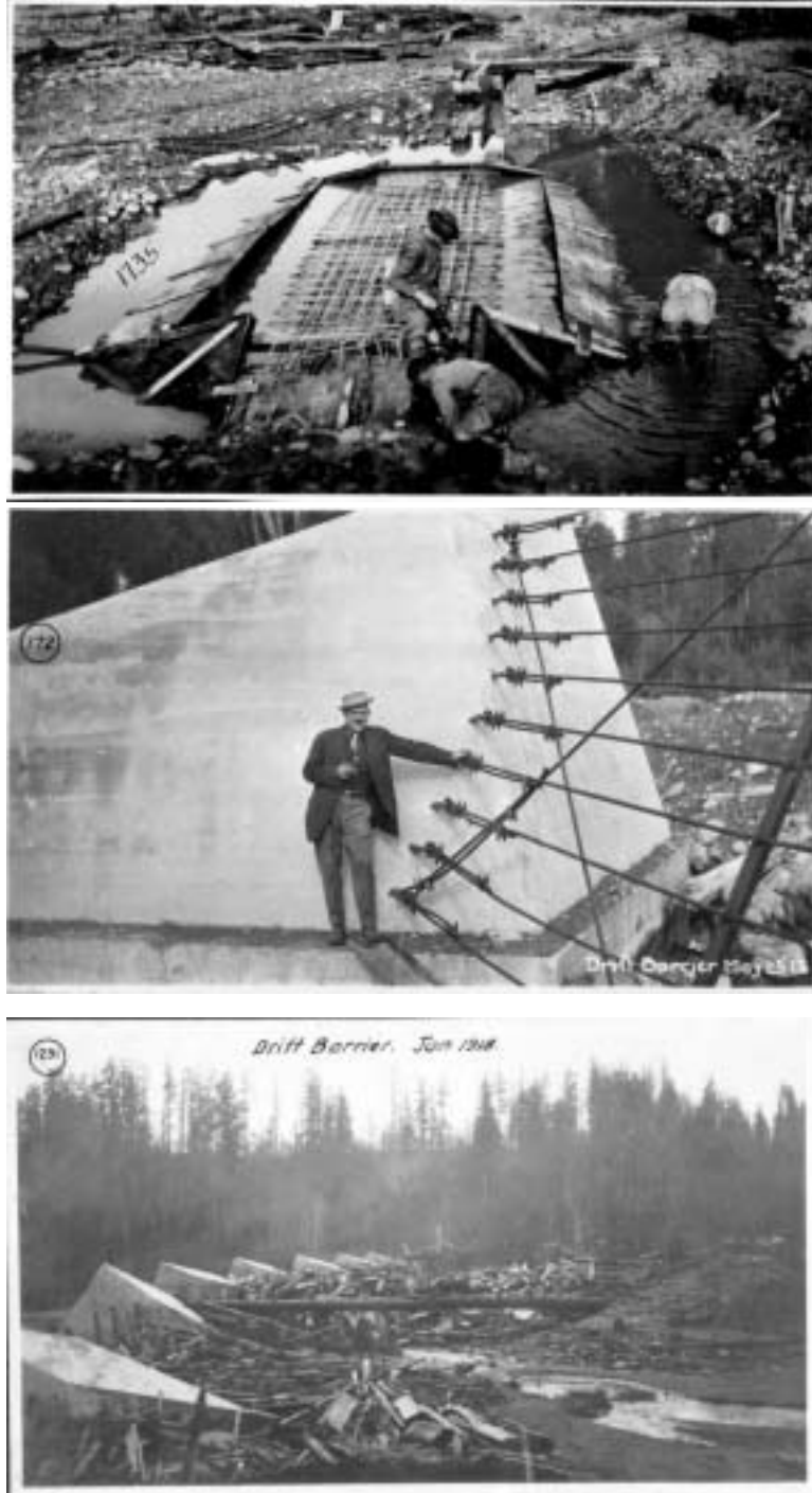
Figure 9. Drift barrier built in 1914 to collect wood upstream of Auburn (see Figure 7 for location). The barrier consisted of a linear series of large concrete blocks anchored in the riverbed with cable strung between. Photos from Inter-County River Improvement District (upper photo undated, probably 1914; middle photo 1915; lower photo 1918).
