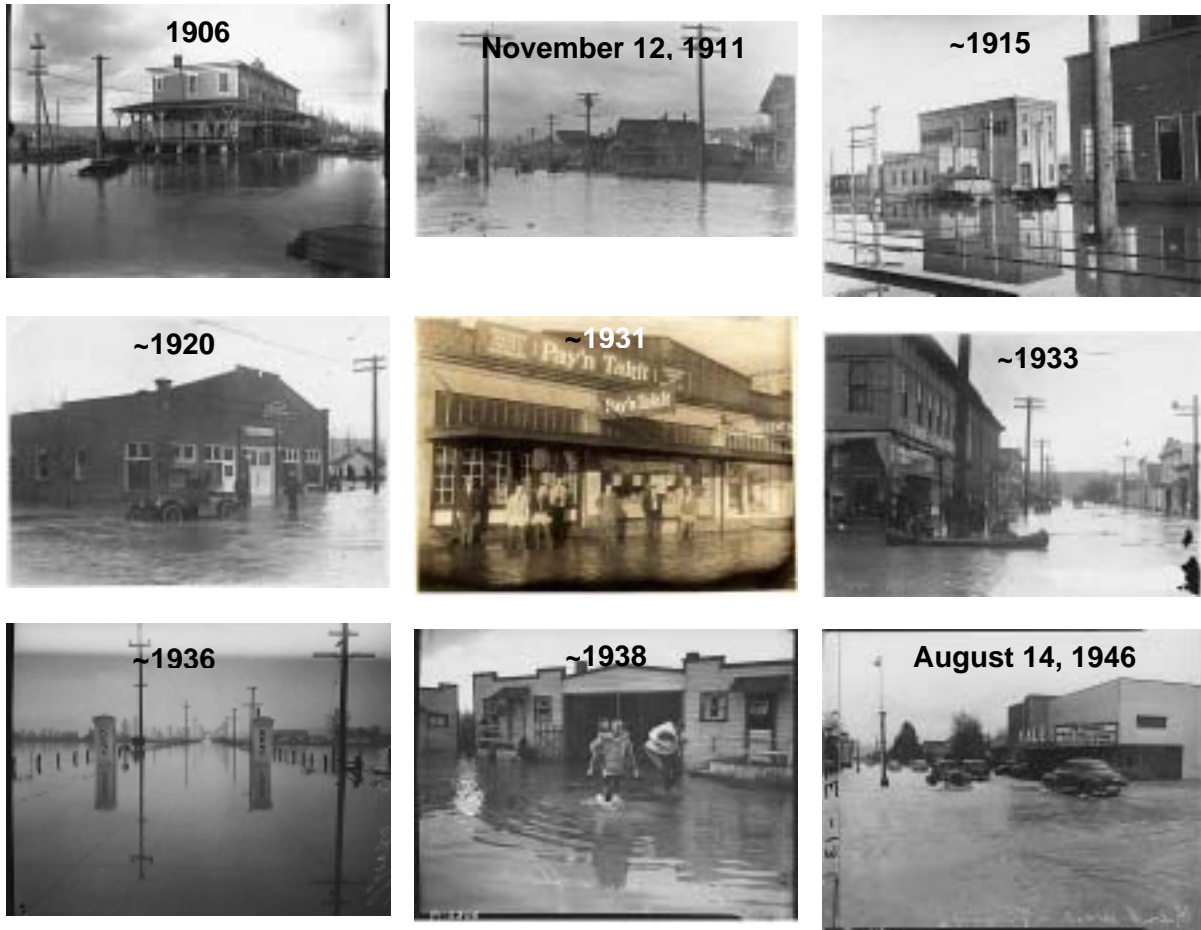
Figure 14. Photographs of flooding in Kent between 1906 and 1946: “Interurban station in a flood, Kent, ca. 1906,” White River Valley Museum Photograph Collection (WRVM) #1161; “Flood in Kent, November 12, 1911,” WRVM #1362; “Kent Interurban Power Station flood, Kent, ca. 1915,” WRVM #55; “Hallock Garage, exterior, during flood, Kent, ca. 1920,” WRVM #922; “Pay’n Takit store in flood, Kent, ca. 1931,” WRVM #3877; “Flood in downtown Kent, ca. 1933,” WRVM #287; “Flooded road at entrance to Kent, 1936,” Museum of History and Industry Photograph Collection (MOHAI) # PI23103; “People leaving flooded house during Green River flood, Kent, 1938,” MOHAI #PI23110; “Flooded street, Kent, August 14, 1946,” MOHAI #PI23132.
