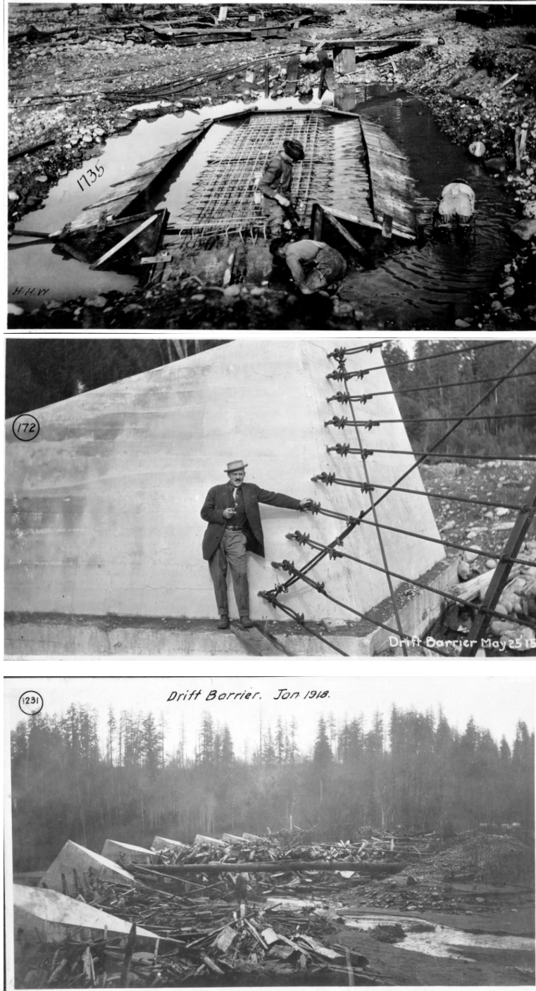
Figure 9. Drift barrier built in 1914 to collect wood upstream of Auburn (see Figure 7 for location). The barrier consisted of a linear series of large concrete blocks anchored in the riverbed with cable strung between. Photos from Inter-County River Improvement District (upper photo undated, probably 1914; middle photo 1915; lower photo 1918).
